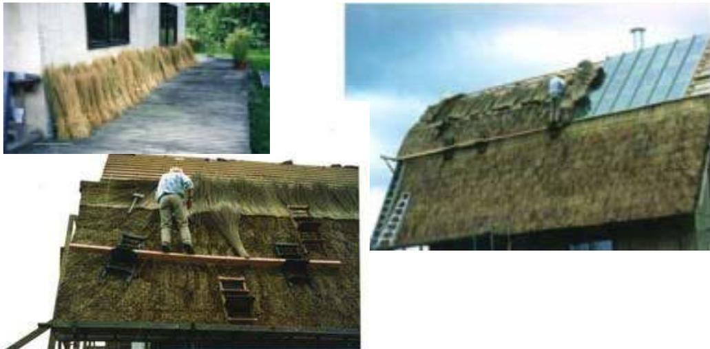
Figure 9 Thatching the roof with bulrush
