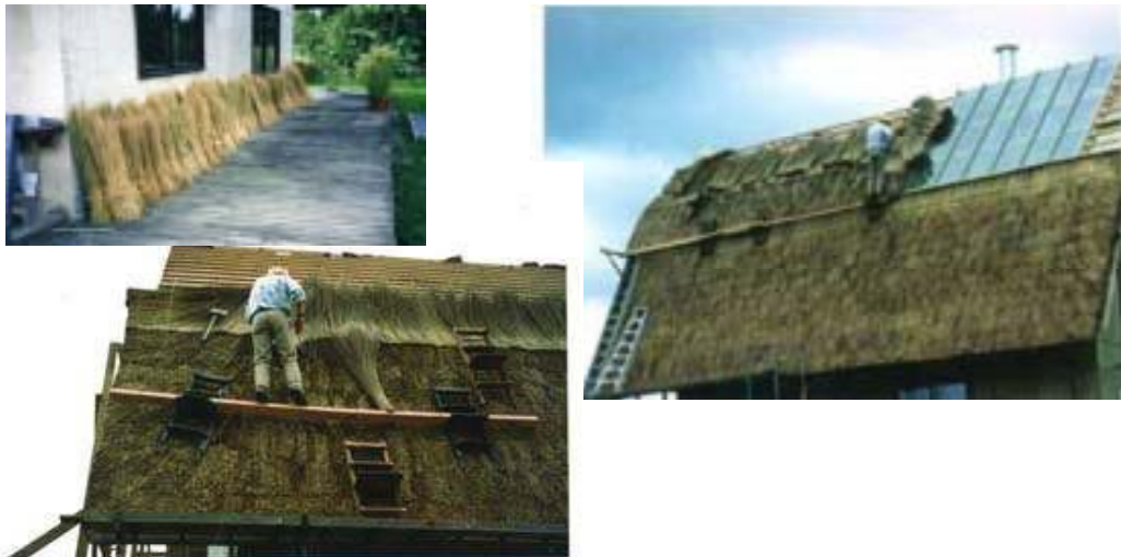
Figure 9 Thatching the roof with bulrush
